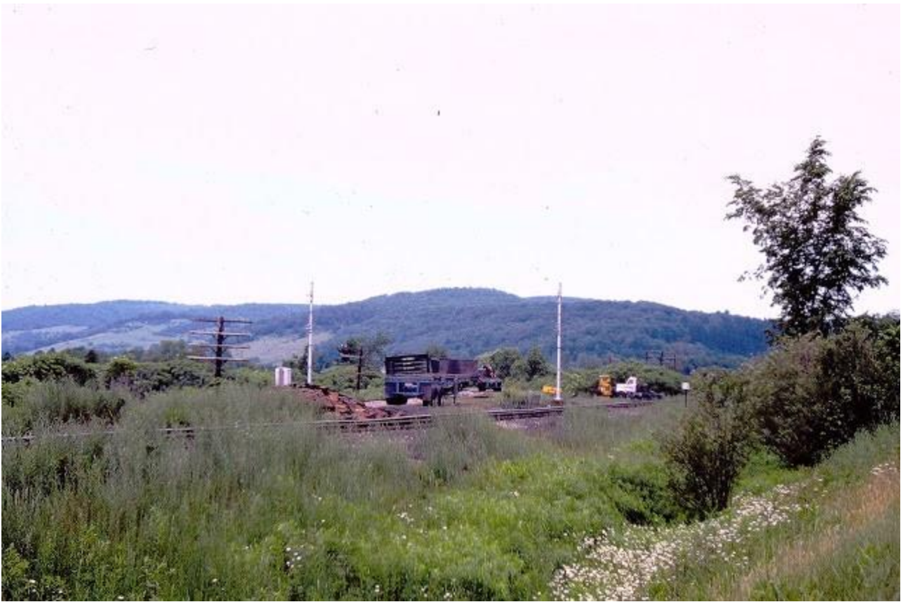
Van Etten Junction during scrapping operations, June 25, 1978 (Paul J. Templeton photograph)
