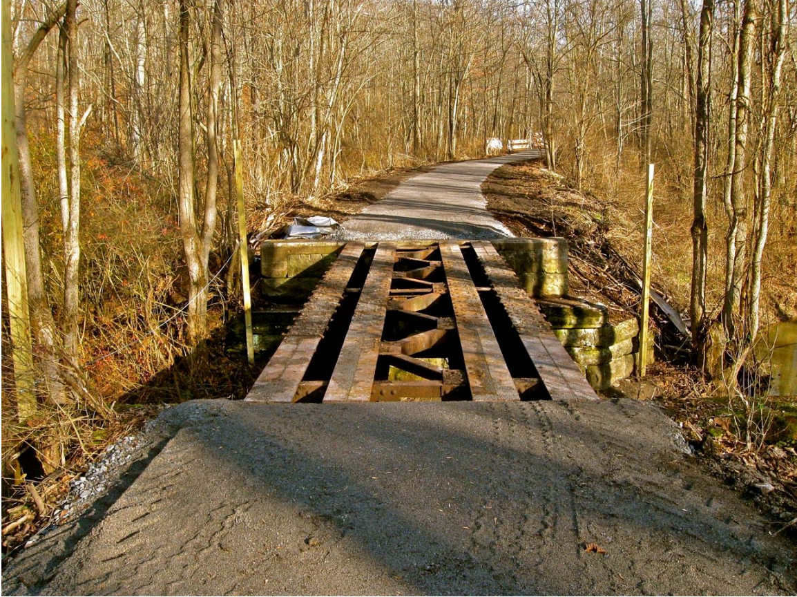
RSY A Bridge
